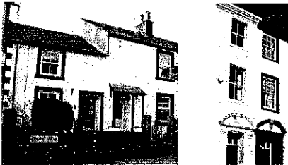
Stone features of pubs and farmhouses are often painted black, but this tends to obscure mouldings in the stone features.
