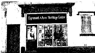
Loss of historic features: pilasters each side of shopfront have been removed and the sign spoils the proportions of the shop window instead of occupying the traditional fascia above.
