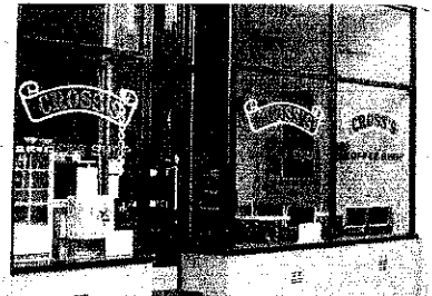
Discrete window signage that does not overwhelm the shopfront and allows full visibility into the premises.
