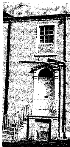
This retrofit foul drainage installation pays no regard to the proportions of this period elevation.
