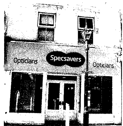
This deep corporate brand sign replaces the original fascia, cornice etc. and destroys the balance of the shopfront.
