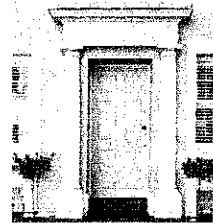
An example of a muted colour, used on a front door.
