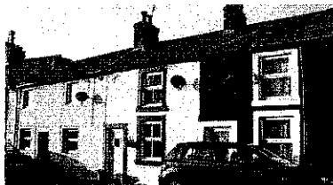
Satellite dishes litter this elevation in a conservation area.
