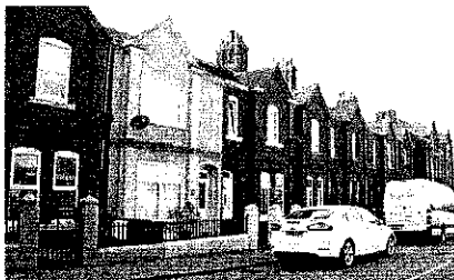
This terrace of houses in Millom is decorated with brick detailing. The second house from the left has been rendered in an inappropriate dash finish burying the brick detailing.
