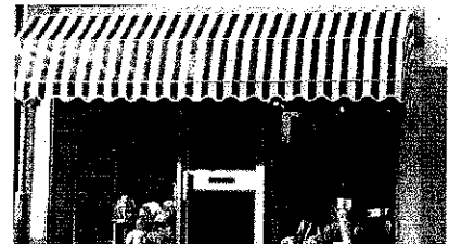
A Dutch awning, although quite attractive, has no historical precedent in a conservation area.
