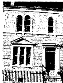
Rusticated finish to ground floor masonry, with deeply incised horizontal lines.
