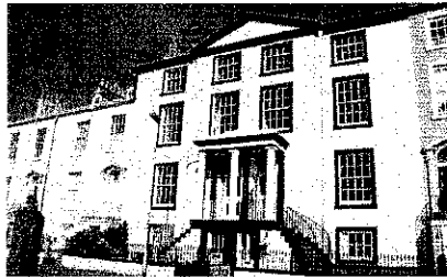
Bold colours, when applied to one part of a unified elevation, can upset its balance.
