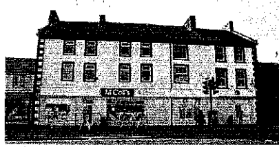
Chimney stacks where pots have been removed appear rather austere.
