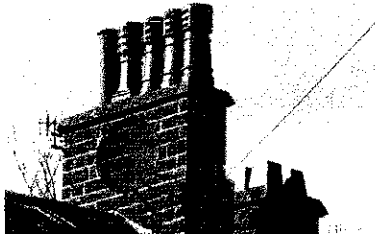
Where possible satellite dishes should be mounted on a rear elevation, but if this is facing the wrong way, then small units can be sited towards the rear of a chimney stack.
