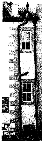
Discretely sited retrofit soil vent pipe, with decorative terminal.
