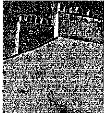
Chimneys stacks on terraces often serve the fireplaces in two houses, so are quite substantial with a large number of pots.
