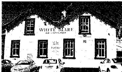
Lettering that is respectful in style and proportion to the elevation in terms of letter style and position.
