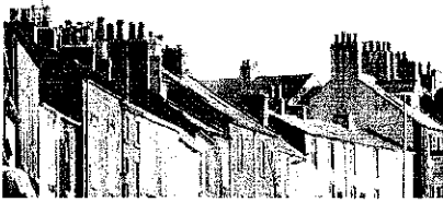
Chimney stacks in St Bees conservation area.
