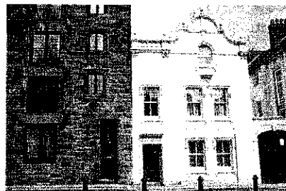
Restored Dutch gabled listed building in Roper Street, Whitehaven, with new windows, external render & refurbished front door.
