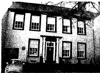
Example of discretely located burglar alarm in corner on side of building.
